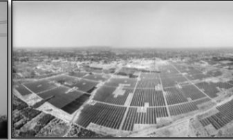
648 MW Ultra Mega Solar Power Plant
