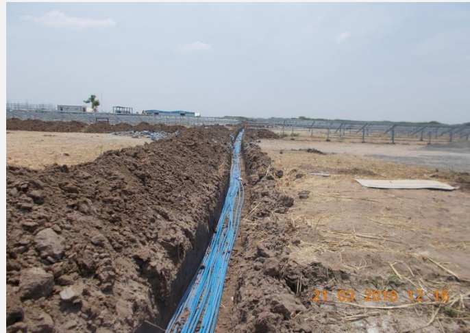
DC Cable Laying & Termination
