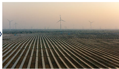
2,140 MW at Jaisalmer, Rajasthan
